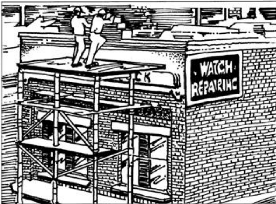
Rehabilitation of block parapet wall.
