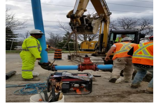
• Cedar Ave. & Palmer Ave. Watermain Replacement
