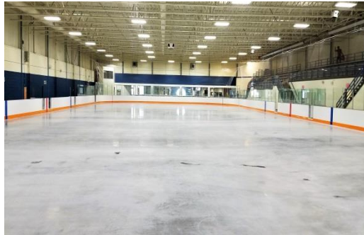
• Elvis Stojko Arena Ice Slab Replacement
