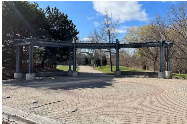
POLYCARBONATE CUT OUT ROOF ALTERATION
