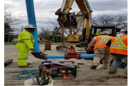
• Cedar Ave. & Palmer Ave. Watermain Replacement
