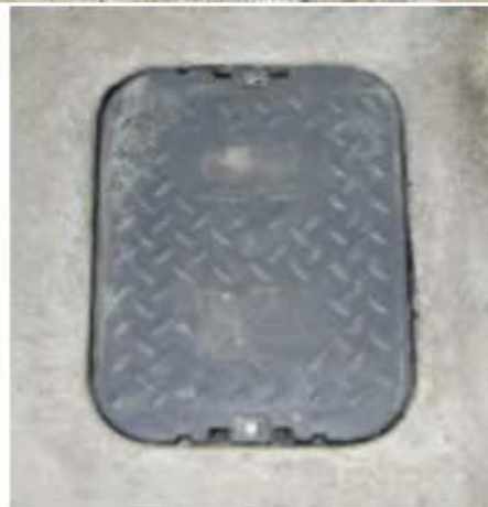
Floor plate cover for backwater valve.
