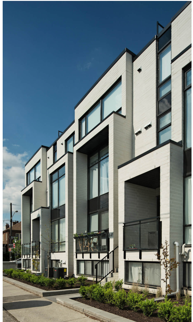
Fig 30: A townhouse with landscaping and raised entrances define private ownership and delineate the semi-private space.
