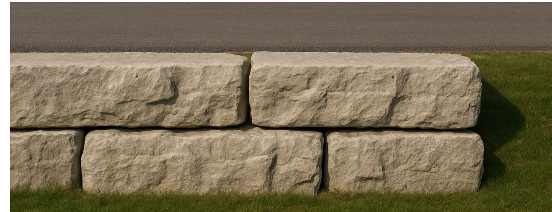
2 ARMOUR STONE RETAINING WALL
